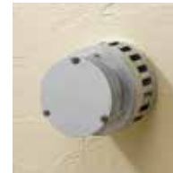
Balanced Flue (No chimney required)
